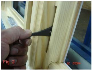
2. Raise lock handle to middle position. At this position, the release tab is most accessible.
