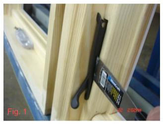
1. Raise lock handle slightly and remove bezel. This can be done simply by hooking a fingernail behind it or prying off with putty knife.
