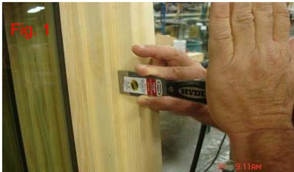
1. Remove sash stops. Starting with the vertical stops, work the thin, stiff putty knife in behind stop, and work loose. Utilizing the small prybar, carefully pry the stops away from jambs so as not to damage them. Remove the horizontal stops in same manner.
