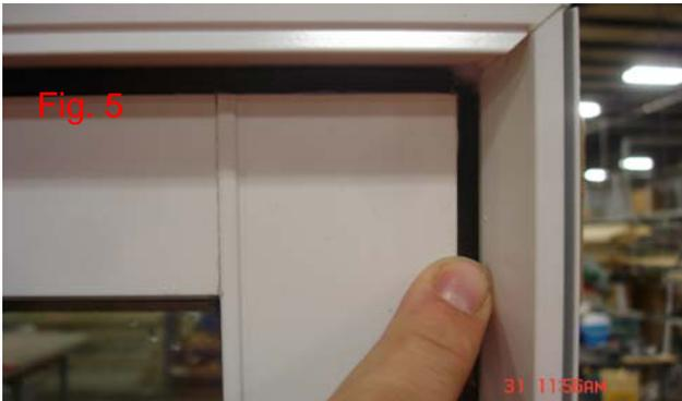
6. Replacement sash can now be installed. This will require a second person, once again. From exterior side, place sash in frame, ensuring that sash is centered. This can be checked by making sure 'reveal' between sash and frame is equal around perimeter of unit. See Fig. 5.
