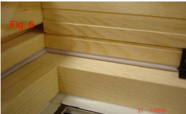
7. Set screws in all four corners of sash brackets, then, again check around sash to make sure reveal is equal, and also check to make sure that the sash is seated against the bulb seal on interior. See Fig. 6. If not, it may be hanging up on one of the centering blocks, and may need to be repositioned. Remainder of sash bracket screws can now be installed.
