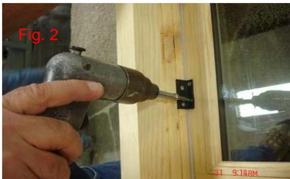
2. Remove screws from bottom portion of clips that hold sash in frame, as shown in fig. 2.
