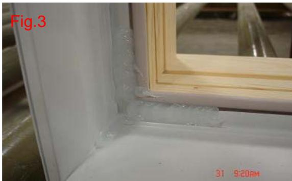
3. Once all screws have been removed and person is staged on exterior of unit, sash can be removed. This is done by applying pressure to each corner, starting at top. Once top corners have 'broken' loose, tilt sash downward. This should help to break caulking loose at bottom corners. You can now remove sash.
