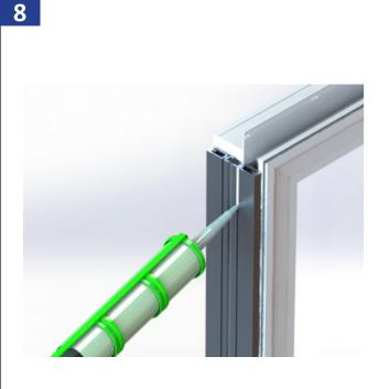
Apply a continuous bead of sealant to the other side of the structural mull groove that will set over the second windows nail fin.
