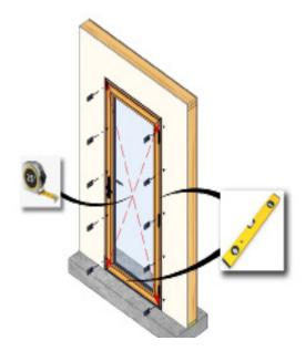
From the interior, square the frame in the opening by installing shims between the jambs and framing. Be sure to block solid behind each hinge.
