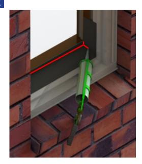
Place a bead of sealant where the existing stool meets the existing window sill.
