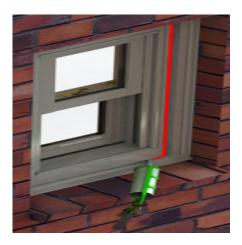
If total frame replacement in brick or siding was preformed maintain a minimum of ¼" between the window frame, trim, siding, or masonry. Apply backer rod (if needed) and a continuous bead of sealant between the window frame and exterior finish material on all four sides of unit. Make sure to clean all surfaces before applying sealant (some surfaces may need to be primed so check with sealant supplier).
