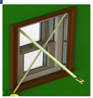
Check for plumb, level, square and window operation. Make any necessary adjustments to shims and finish installing frame screws. Raise bottom sash to install bottom screws, and tilt bottom sash in to install center screws.
