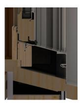
Cut the sill adapter to the correct height. Use a sharp utility knife to score the sill adapter along the groove. Bend and break off the excess sill adapter material and install on window
