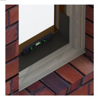
Check the sill for level or for bowing and shim as needed to level sill. Place shims about ½" from each side and in center with minimum spacing of 16". Attach shims to prevent movement after they are level.
